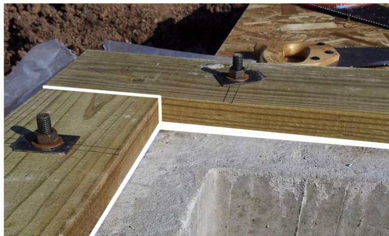
Figure 1-3. Sill Plate Installation.
