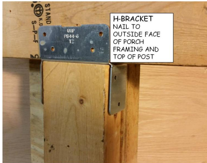
Figure 6-2. Porch Post H-Bracket.
