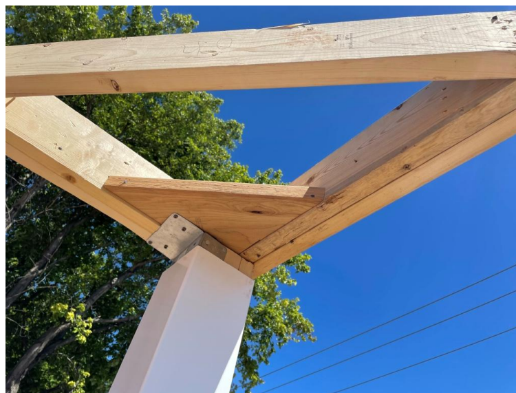
Figure 6-3. Porch Post Trim Ring Blocking.
