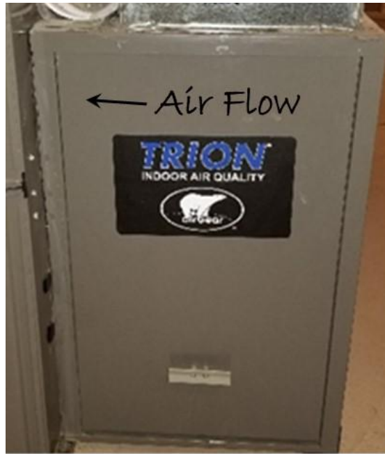
Figure 21-1. Furnace Air Flow Direction.
