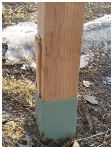
Figure 20-4. Installation of Mailbox Post.
