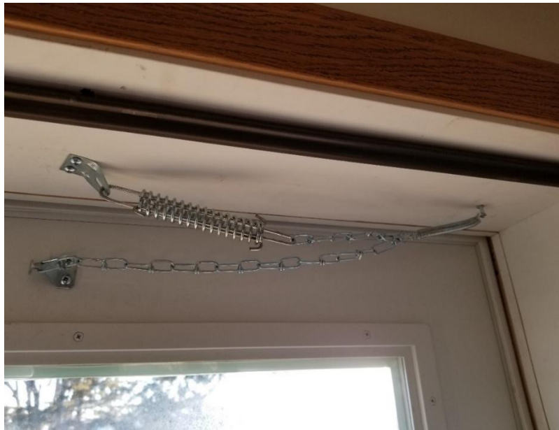
Figure 20-1. Storm Door Wind Chain.
