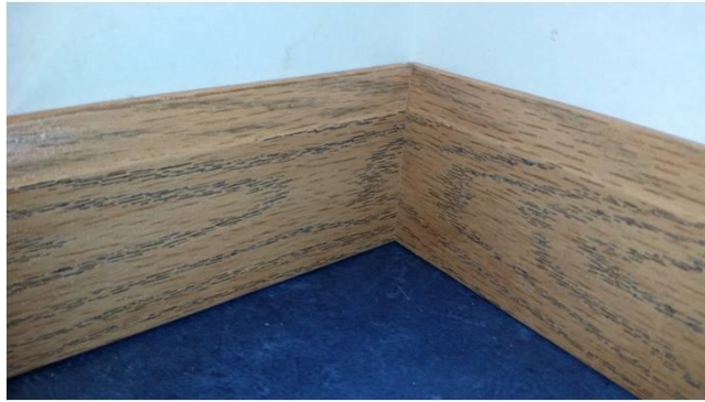
Figure 19-9. Finished Coped Joint.
