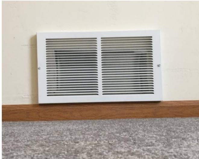
Figure 19-12. Positioning Cold Air Return Vent Covers.
