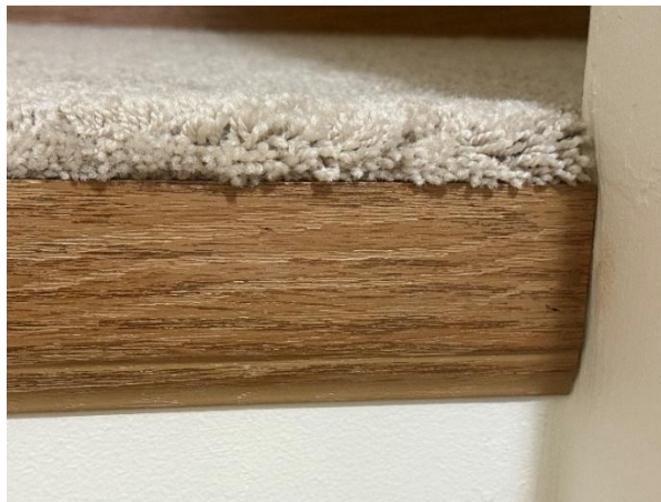
Figure 19-2. Closet Platform Edge Trim After Carpet Installation.
