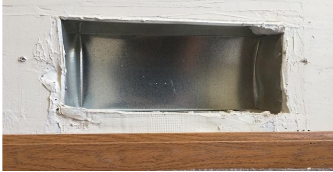
Figure 19-11. Sealing Plaster Gaps Around Cold Air Returns
