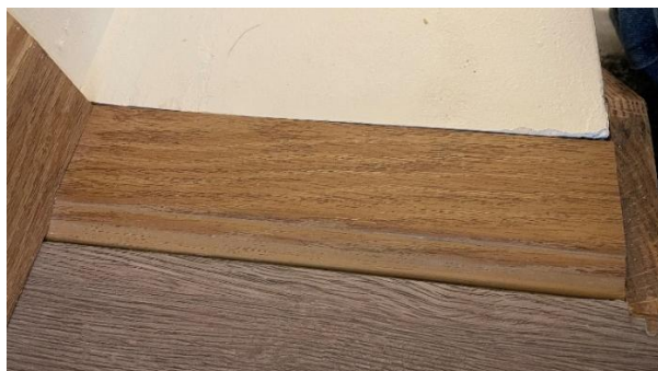
Figure 19-3. Stairway Trim Finish With Ledge.
