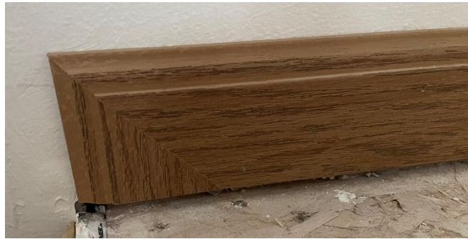
Figure 19-1. Trim End Finish in Closet Platform.
