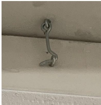
Figure 19-13. Garage Scuttle Cover Hook and Eye Assembly.
