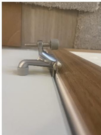
Figure 18-1. Correct Bumper Orientation.
