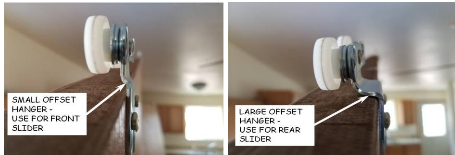
Figure 18-2. Sliding Door Hangers.
