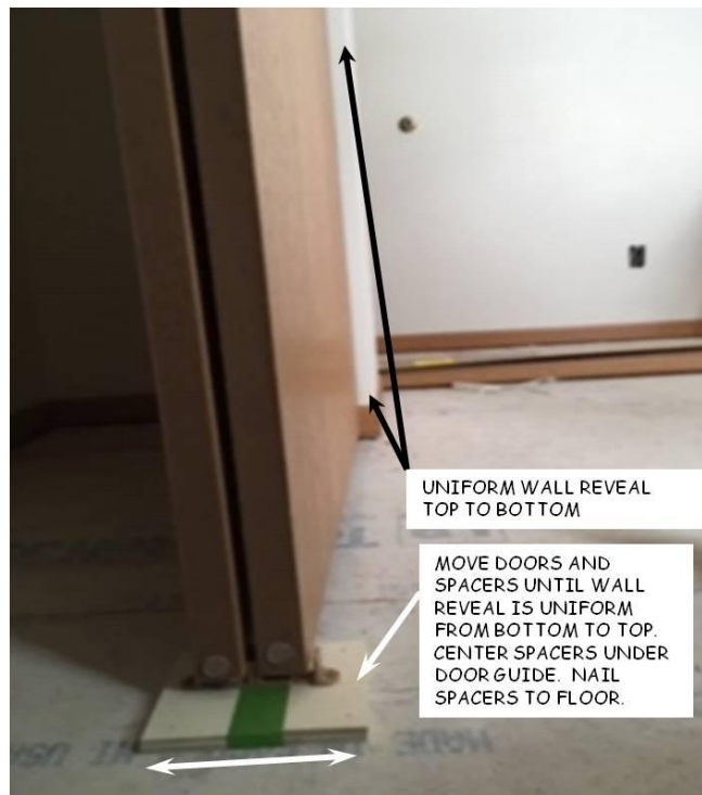
Figure 18-5. Shim Adjustment for Uniform Door Reveal.
