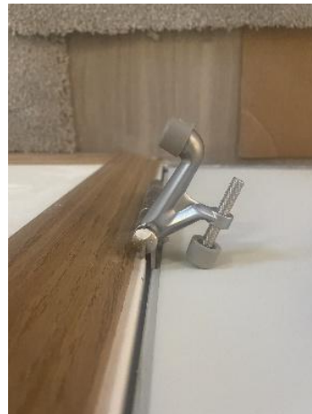
Incorrect Bumper Orientation.
