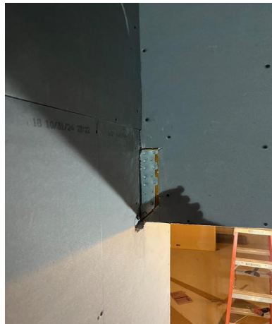
Figure 14-7. Trimming Around Joist Hangers.
