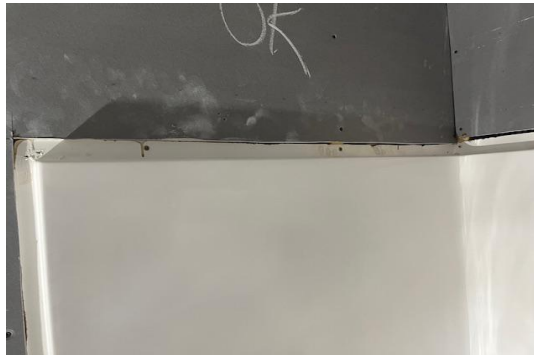
Figure 14-10. Sheetrocking Around Tub/Shower Nailing Flange.
