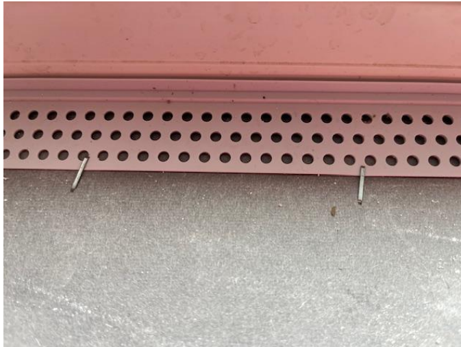
Figure 14-9. Final Staple Securement of Edging Strips.
