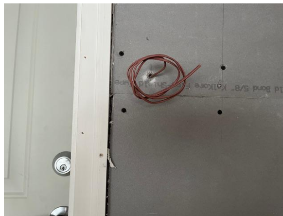
Figure 14-6. Pulling Wires Through Sheetrock.
