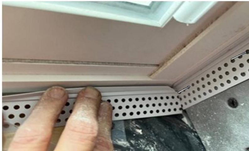
Figure 14-8. 45° Clipped Corners and Inside Row Hole Stapling.
