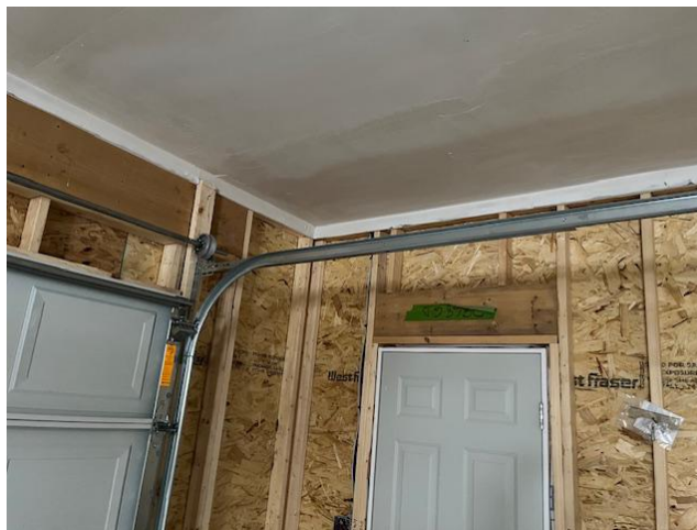
Figure 13-6. Covering Garage Exterior Wall Plates.
