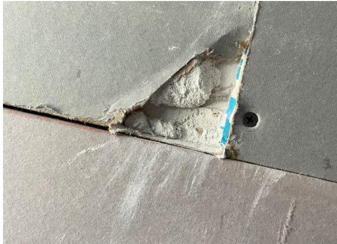
Figure 13-2. Broken Corner.
