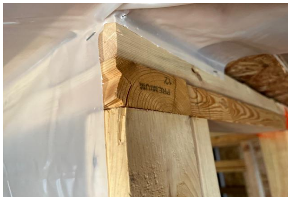
Figure 12-10. Extending Poly Around a Corner.
