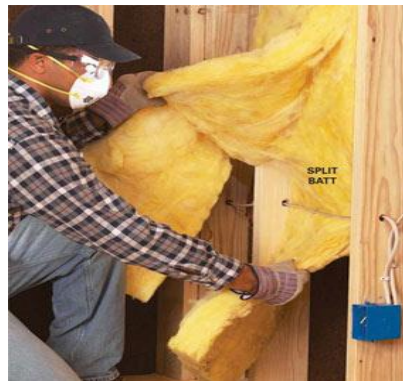
Figure 12-7. Insulating Around Electrical Wires.
