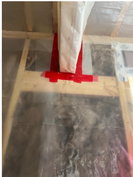
Figure 12-12 Air Sealing Around a Flush Closet Header.
