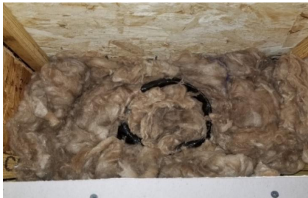
Figure 12-2. Insulation Filled Around Future Fan Vent Duct.
