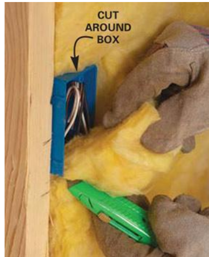
Figure 12-8. Insulating Around Electrical Box.
