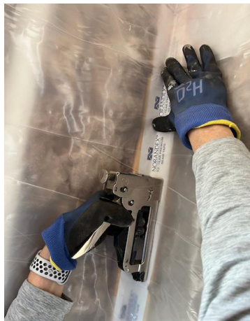
Figure 12-11. Pushing Poly Into The Corner While Stapling.
