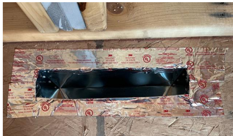
Figure 12-4. Sealing In-Floor Heating Duct.
