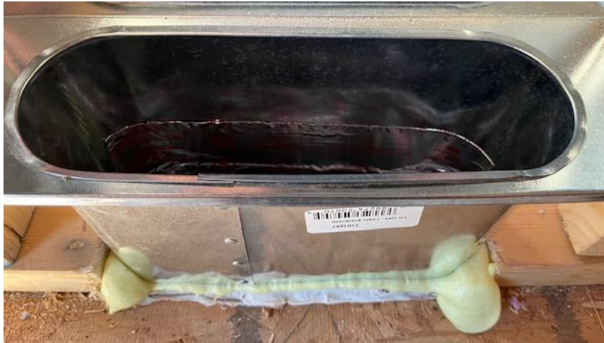
Figure 12-5. Sealing Cold Air Return Joints
