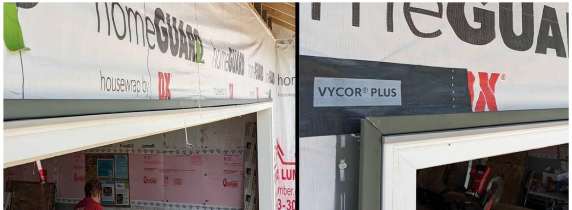
Figure 11-15. Housewrap Over OHD.
