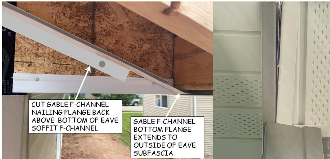
Figure 11-6. F-Channel at Gable Corner.
