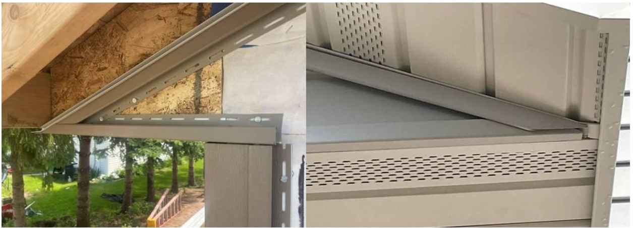
Figure 11-8. J-Channel at Gable Corner.
