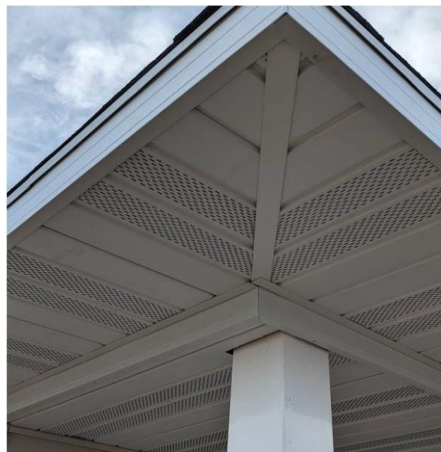
Figure 11-24. Porch Soffit Corner.
