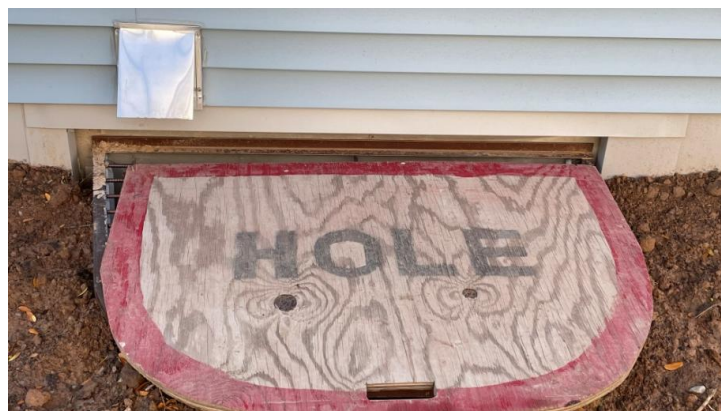
Figure 11-3. Skirting Around Egress Window.
