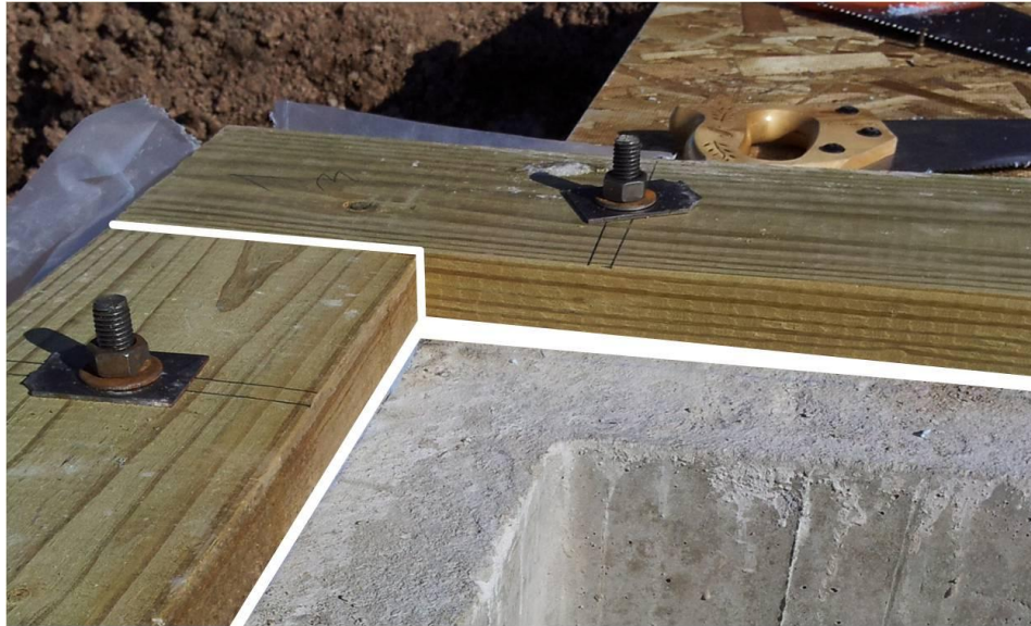
Figure 1-3. Sill Plate Installation.
