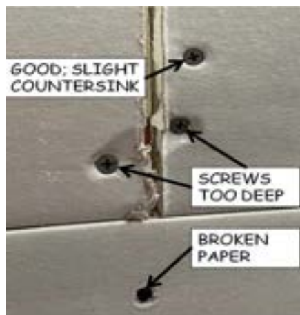
Figure 14-1. Examples of Countersunk Sheetrock Screws.
