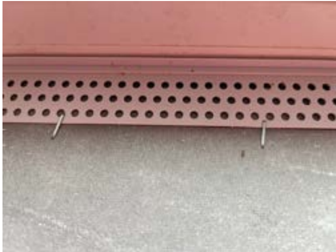
Figure 14-9. Final Staple Securement of Edging Strips.
