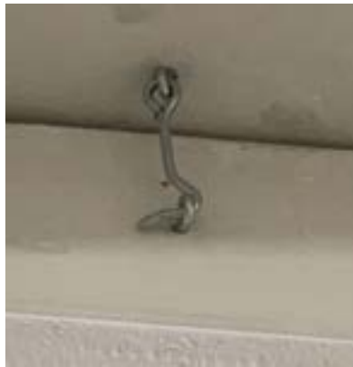
Figure 19-13. Garage Scuttle Cover Hook and Eye Assembly.
