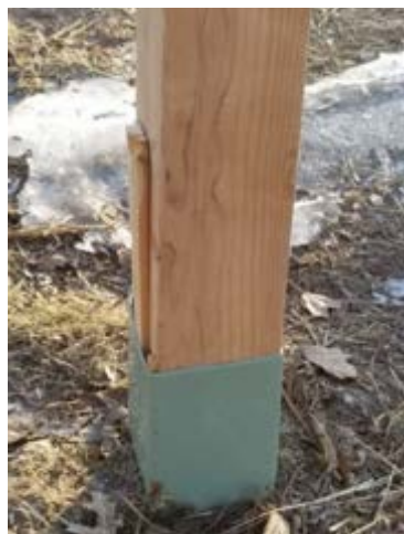
Figure 20-4. Installation of Mailbox Post.
