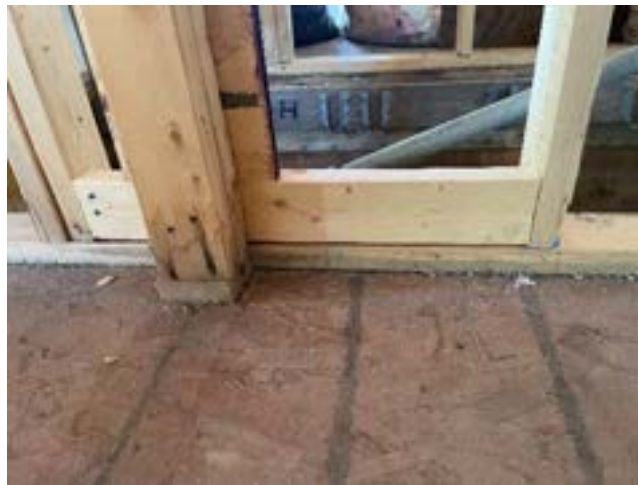
Figure 10-9. Closet Wall Blocking.
