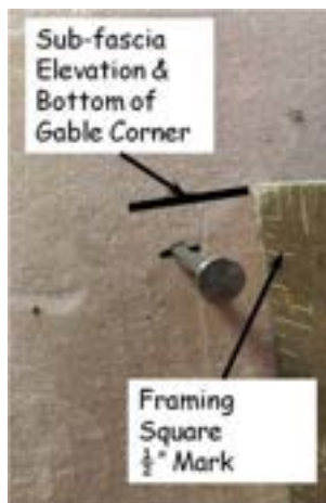
Figure 11-1. Siding Layout.
