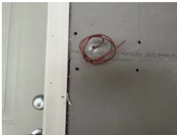
Figure 14-6. Pulling Wires Through Sheetrock.
