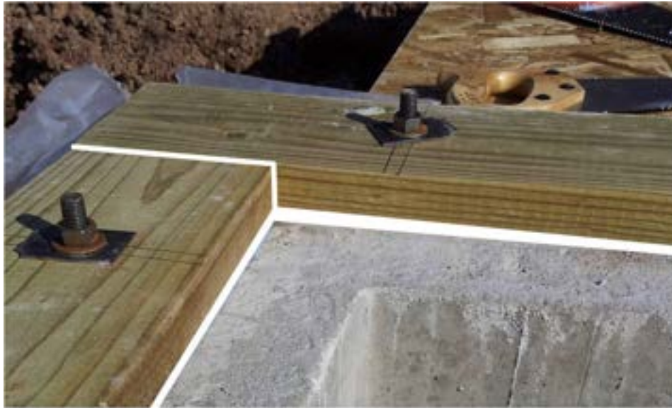
Figure 1-3. Sill Plate Installation.
