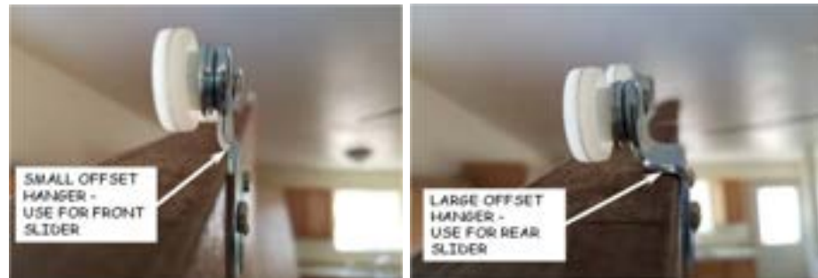
Figure 18-2. Sliding Door Hangers.
