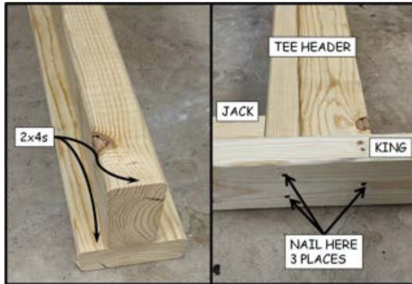
Figure 4-3. T-Header Assembly.
