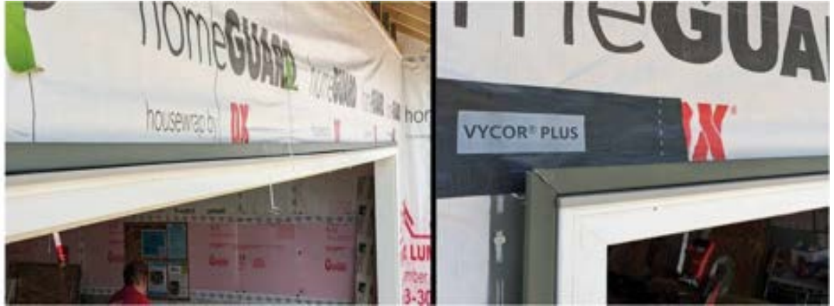
Figure 11-15. Housewrap Over OHD.
