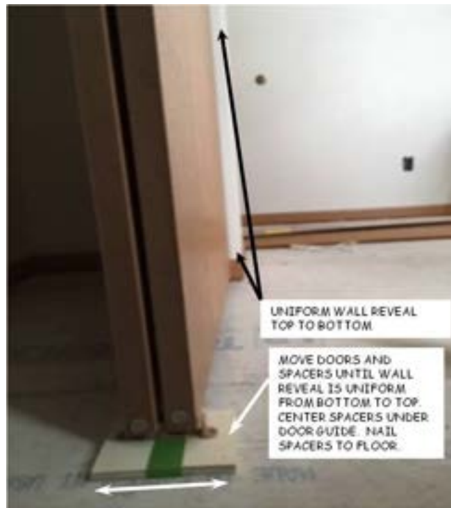
Figure 18-5. Shim Adjustment for Uniform Door Reveal.
