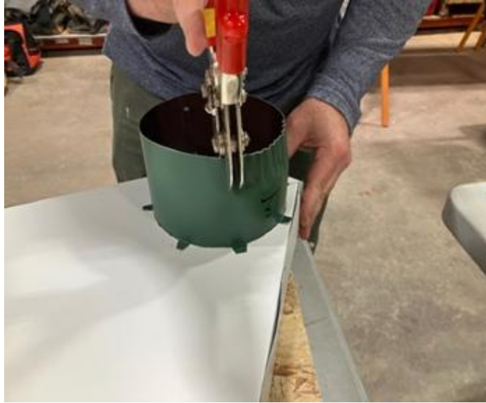
Figure C-17. Crimping Exhaust Pipe.
