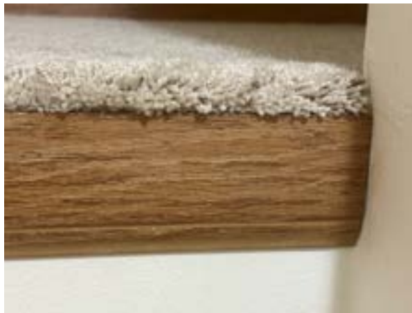
Figure 19-2. Closet Platform Edge Trim After Carpet Installation.
