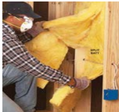
Figure 12-7. Insulating Around Electrical Wires.
