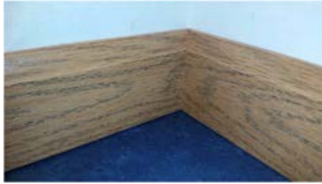
Figure 19-9. Finished Coped Joint.
