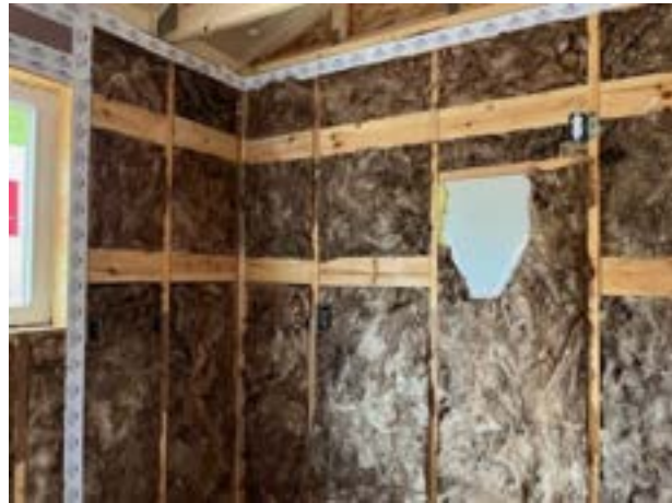
Figure 10-4. Kitchen Cabinet Blocking
