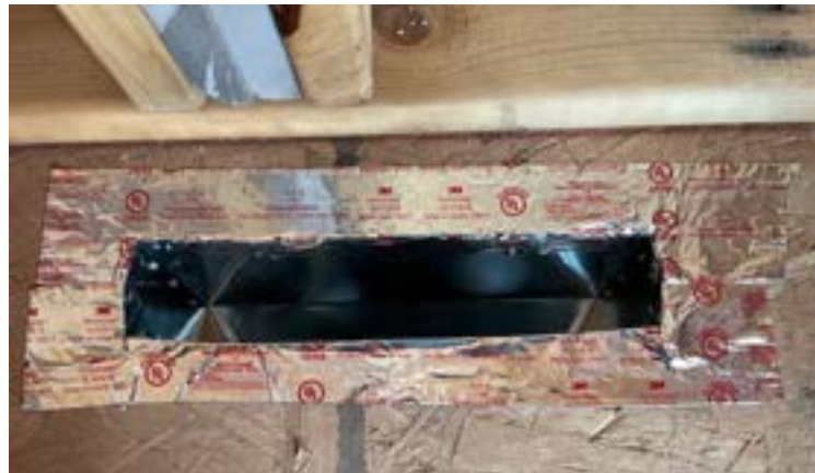
Figure 12-4. Sealing In-Floor Heating Duct.
