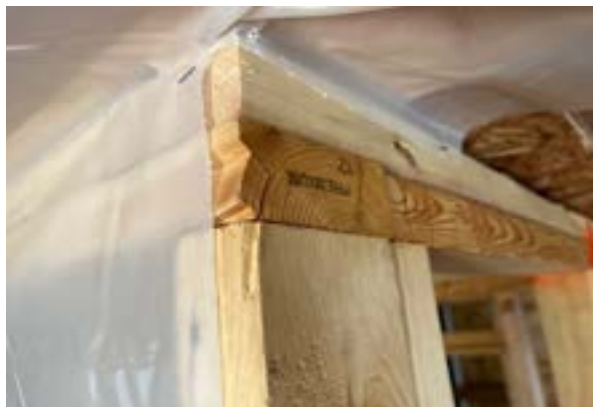
Figure 12-10. Extending Poly Around a Corner.
