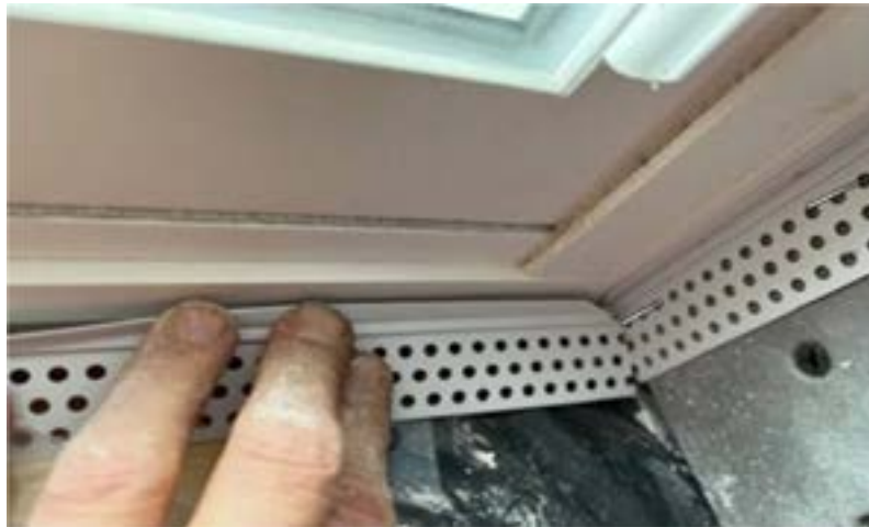
Figure 14-8. 45° Clipped Corners and Inside Row Hole Stapling.
