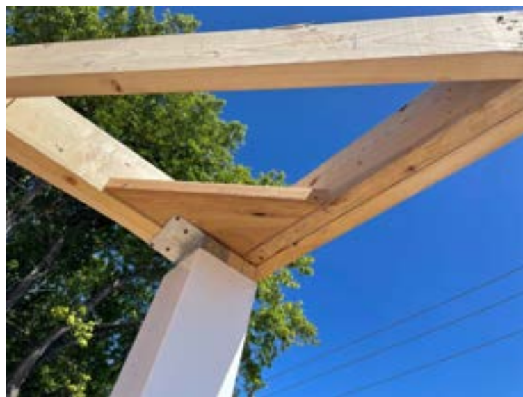
Figure 6-3. Porch Post Trim Ring Blocking.
