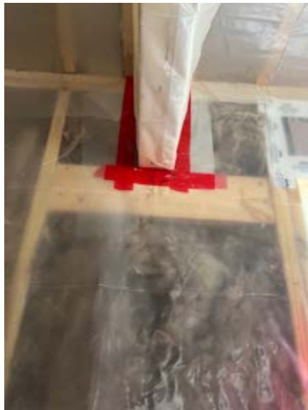
Figure 12-12 Air Sealing Around a Flush Closet Header.
