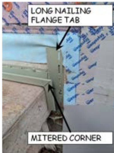
Figure 11-13. Porch Slab J-Channel.
