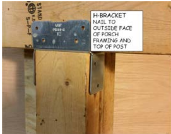
Figure 6-2. Porch Post H-Bracket.
