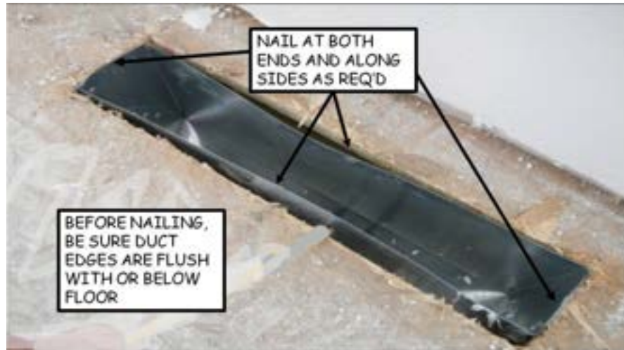
Figure 12-3. Securing In-Floor Heating Duct.
