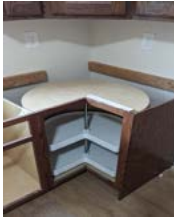
Figure 17-3. Showing Countertop 2x4 Corner Supports.
