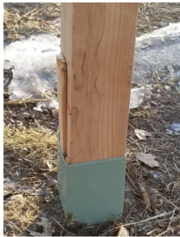
Figure 20-3. Installation of Mailbox Post.
