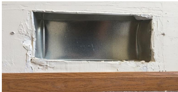
Figure 19-7. Sealing Plaster Gaps Around Cold Air Returns
