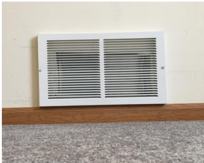
Figure 19-8. Positioning Cold Air Return Vent Covers.
