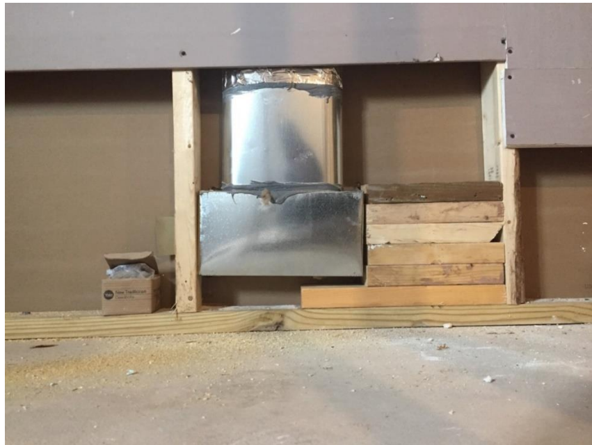
Figure 10-7. Cold Air Return Blocking.
