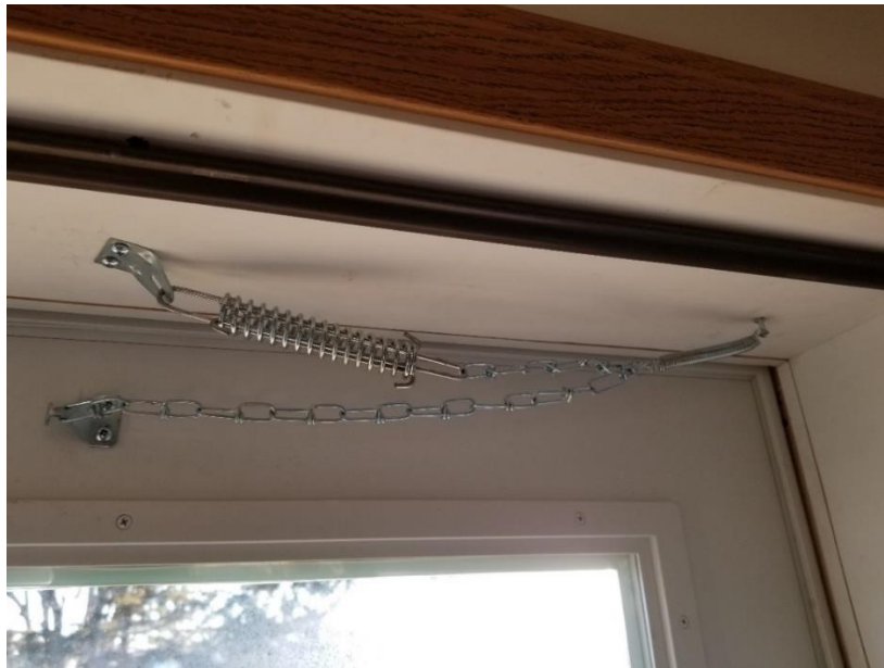
Figure 20-1. Storm Door Wind Chain.
