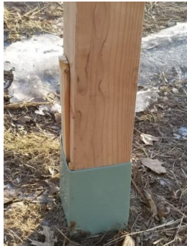
Figure 20-3. Installation of Mailbox Post.
