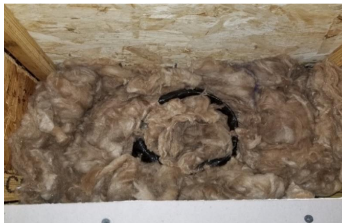
Figure 12-2. Insulation Filled Around Future Fan Vent Duct.
