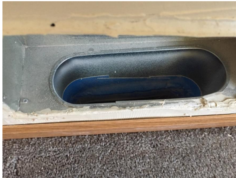
Figure 12-5. Sealing Cold Air Return Joints
