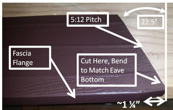
Figure 11-16. Eave End Gable Fascia.
