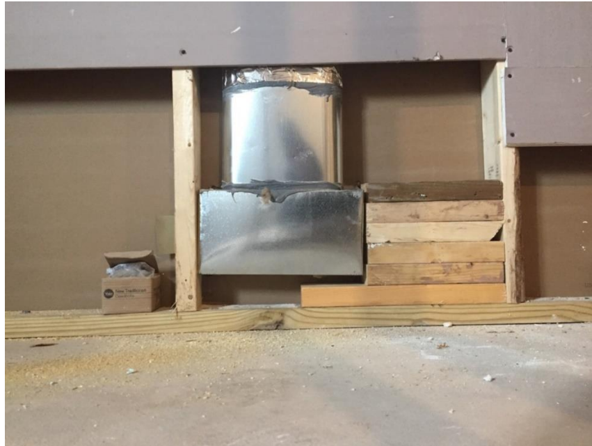
Figure 10-7. Cold Air Return Blocking.
