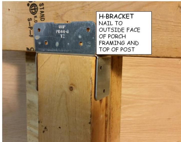
Figure 6-2. Porch Post H-Bracket.
