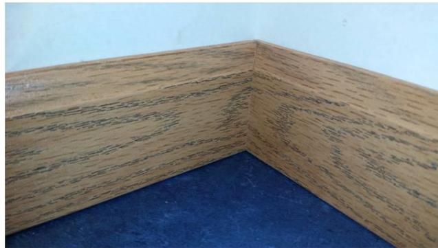
**Figure 19-5. Finished Coped Joint.**
