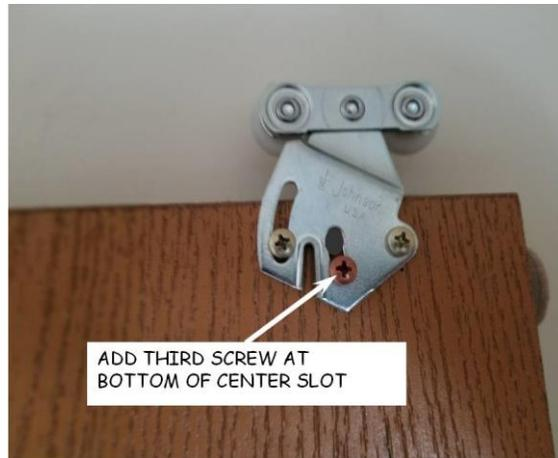
**Figure 18-3. Closet Door Hanger with 3<sup>rd</sup> Screw Installed.**
