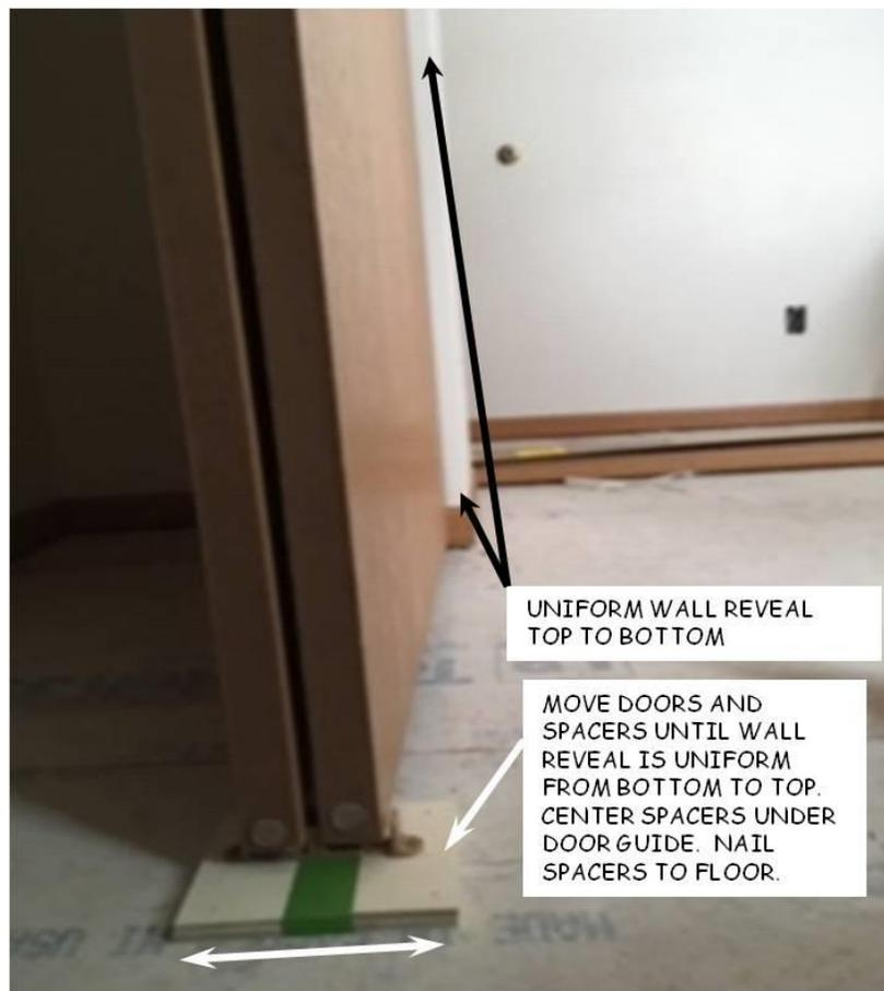
**Figure 18-4. Spacer Adjustment for Uniform Door Reveal.**
