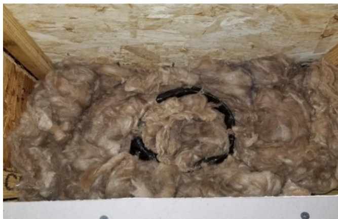
Figure 12-2. Insulation Filled Around Future Fan Vent Duct.
