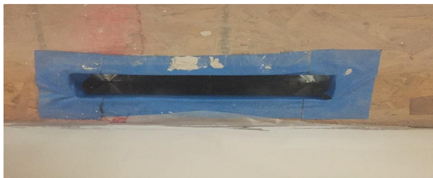
Figure 12-4. Sealing In-Floor Heating Ducts
