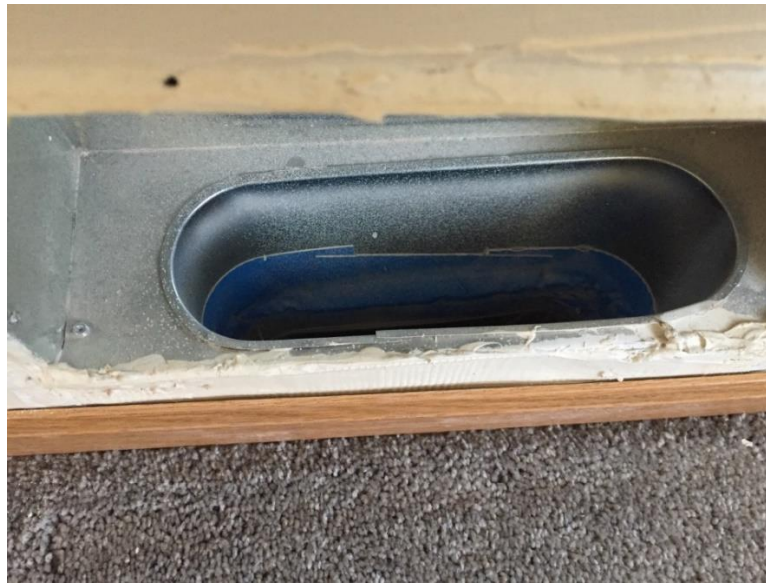
Figure 12-5. Sealing Cold Air Return Joints
