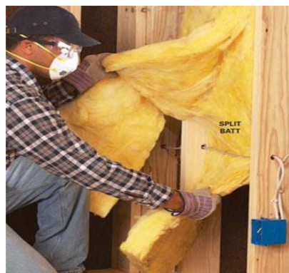
Figure 12-6. Insulating Around Electrical Wires.
