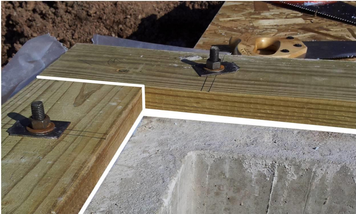
Figure 1-3. Sill Plate Installation.
