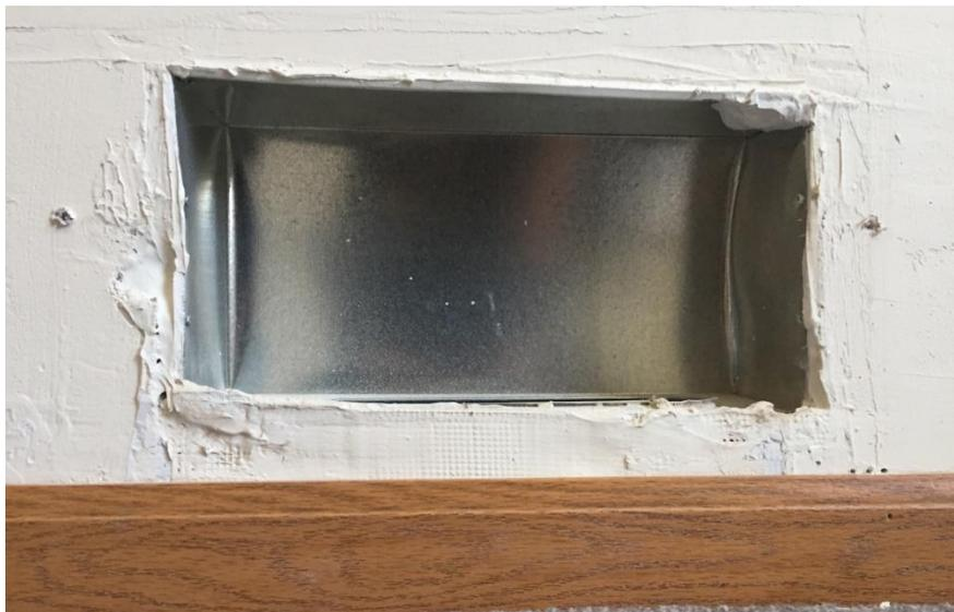
**Figure 19-7. Sealing Plaster Gaps Around Cold Air Returns**
