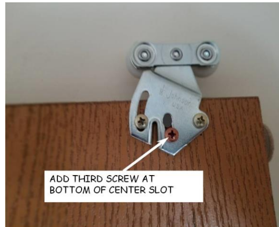
Figure 18-3. Closet Door Hanger with 3 rd Screw Installed.
