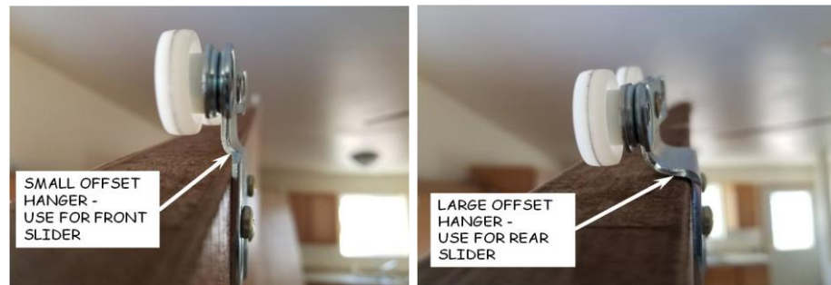
Figure 18-1. Sliding Door Hangers.
