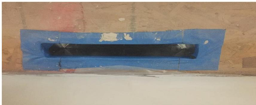
**Figure 12-4. Sealing In-Floor Heating Ducts**
