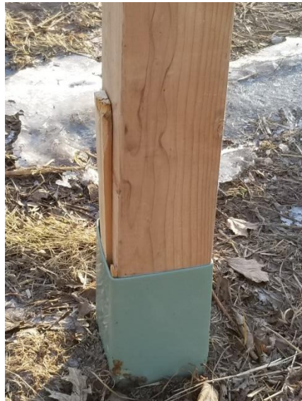
Figure 20-2. Installation of Mailbox Post.
