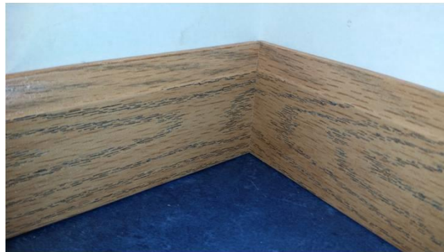
Figure 19-5. Finished Coped Joint.
