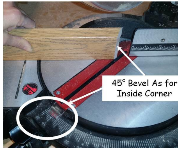
Figure 19-1. Base Trim Bevel Cut.
