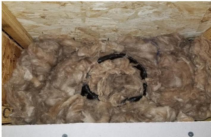
**Figure 12-2. Insulation Filled Around Future Fan Vent Duct.**
