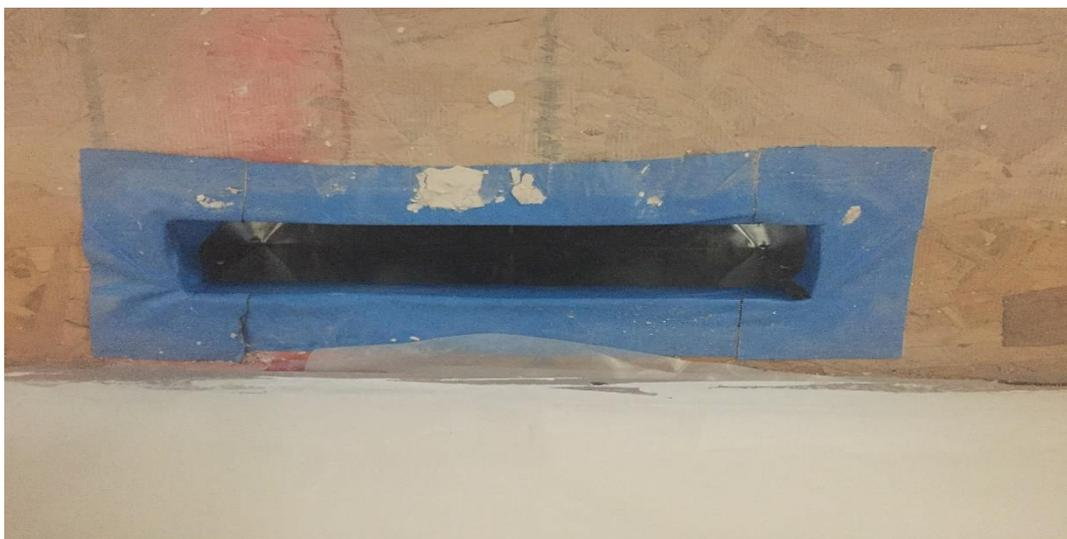
**Figure 12-4. Sealing In-Floor Heating Ducts**
