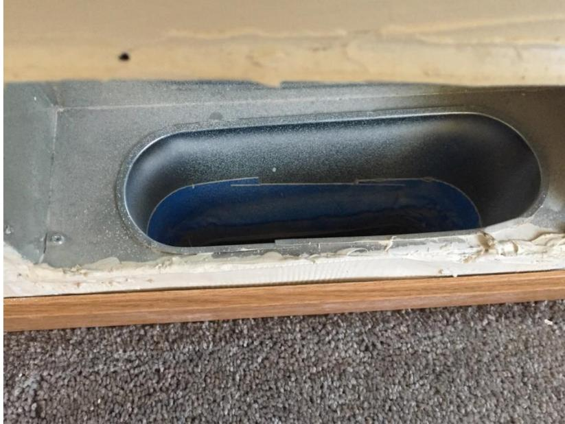
**Figure 12-5. Sealing Cold Air Return Joints**
