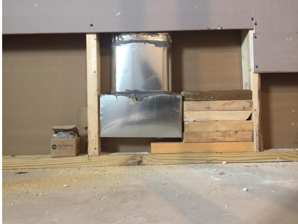
Figure 10-7. Cold Air Return Blocking.
