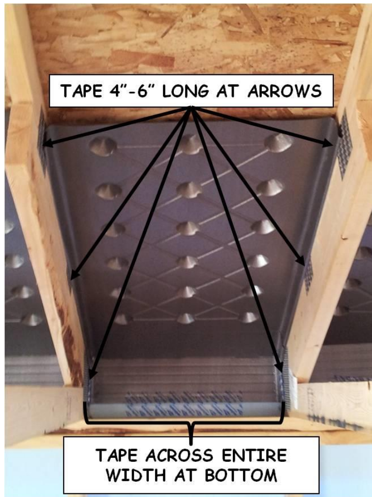
Figure 10-2. Proper Vent Installation.
