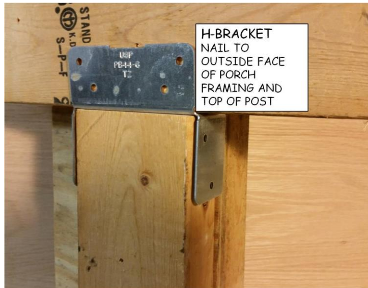
Figure 6-3. Porch Post H-Bracket.
