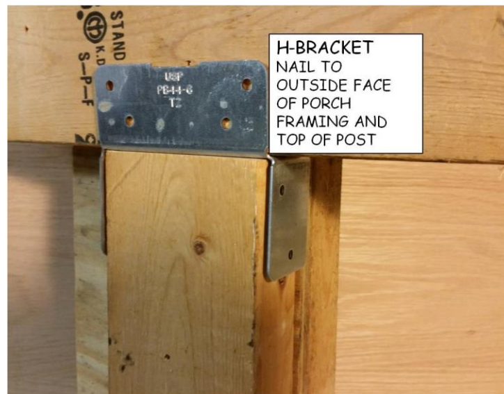
Figure 6-3. Porch Post H-Bracket.
