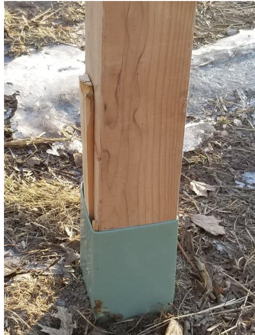
Figure 20-2. Installation of Mailbox Post.
