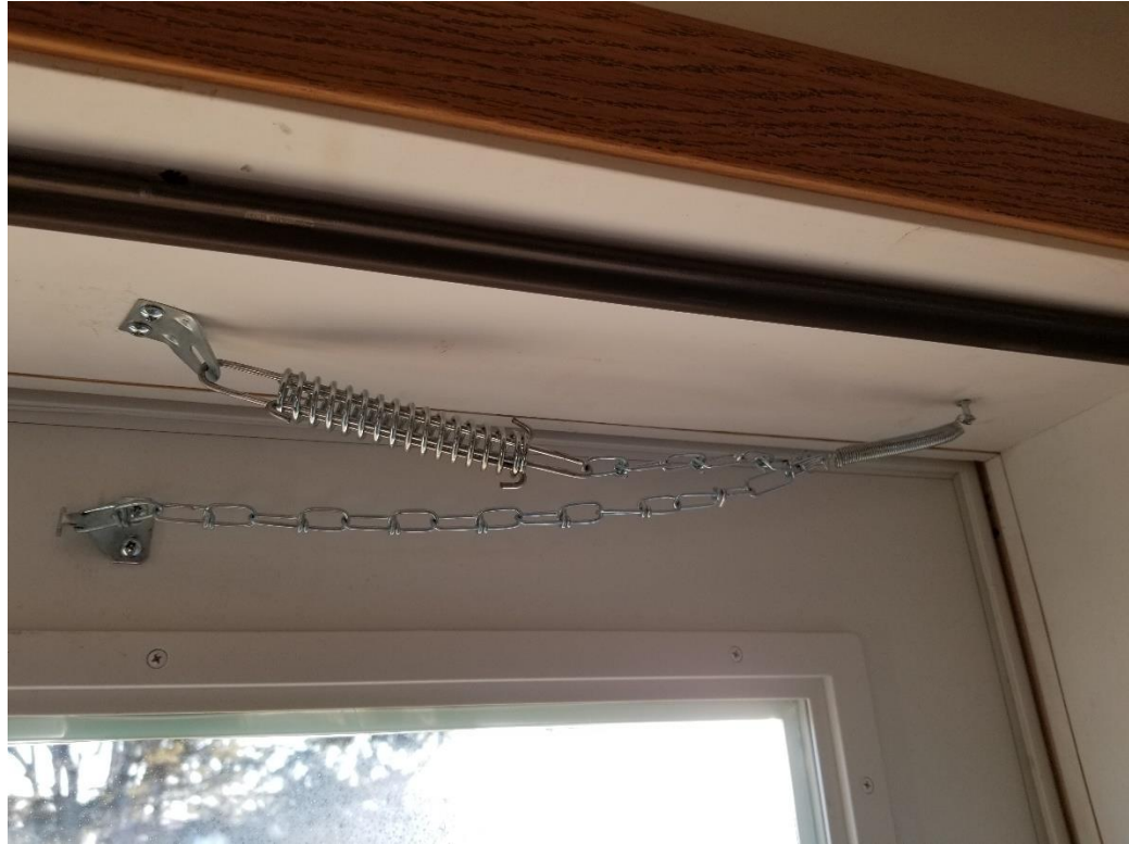
Figure 20-1. Storm Door Wind Chain.
