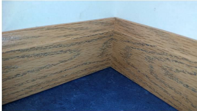
Figure 19-6. Finished Coped Joint
