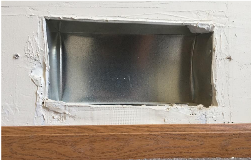
Figure 19-8. Sealing Plaster Gaps Around Cold Air Returns
