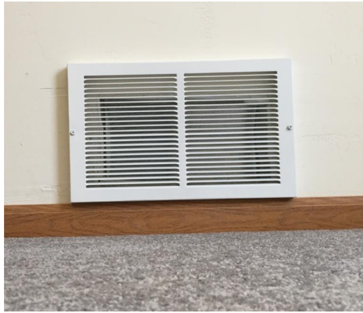
Figure 19-9. Positioning of Cold Air Returns.
