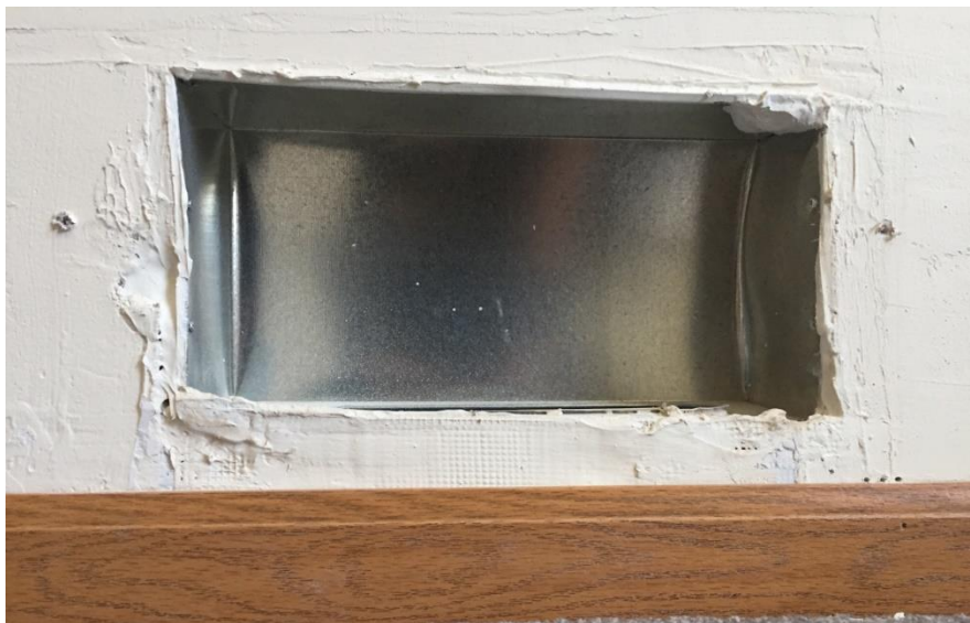
Figure 19-7. Sealing Plaster Gaps Around Cold Air Returns
