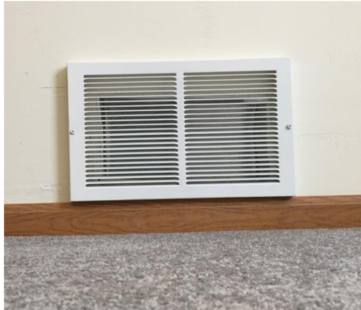
Figure 19-8. Positioning of Cold Air Returns.
