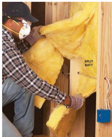
Figure 12-4. Insulating Around Electrical Wires.
