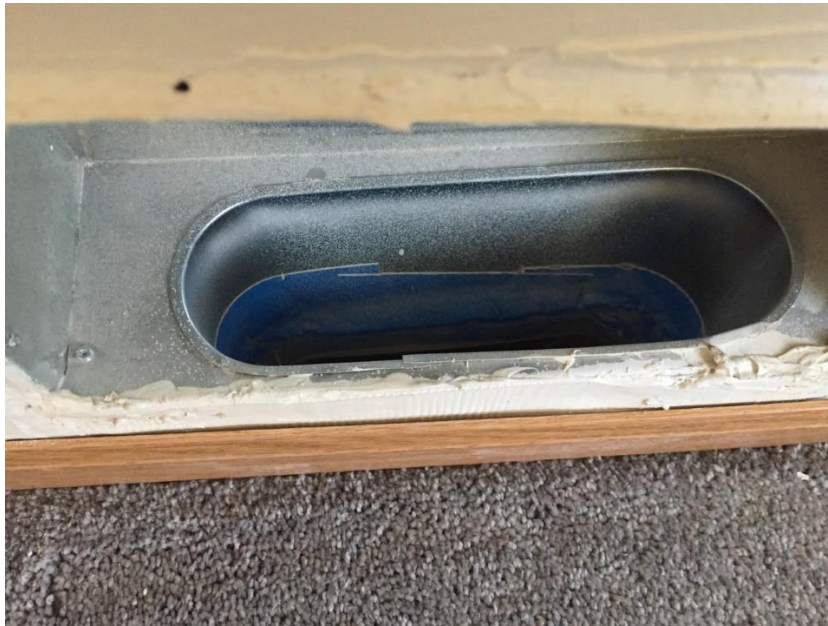
Figure 12-5. Sealing Cold Air Return Joints
