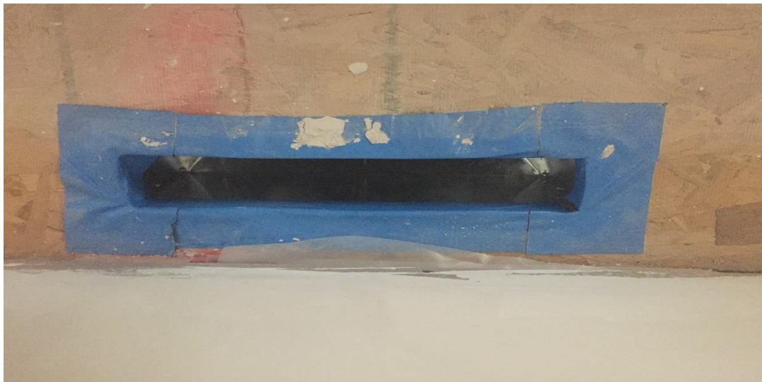
Figure 12-4. Sealing In-Floor Heating Ducts
