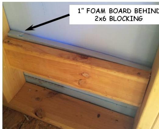
Figure 11-1. 2x6 Blocking for J-blocks.
