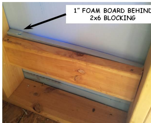
Figure 11-1. 2x6 Blocking for J-blocks.
