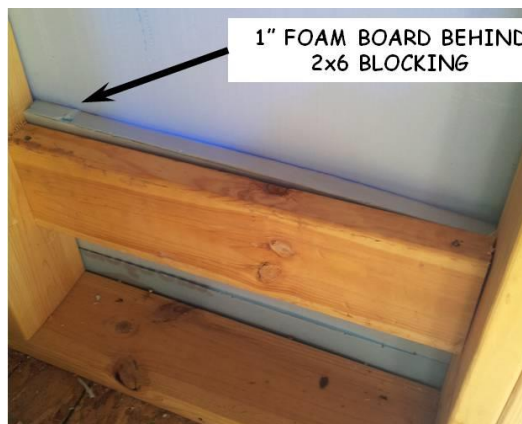
Figure 11-1. 2x6 Blocking for J-blocks.
