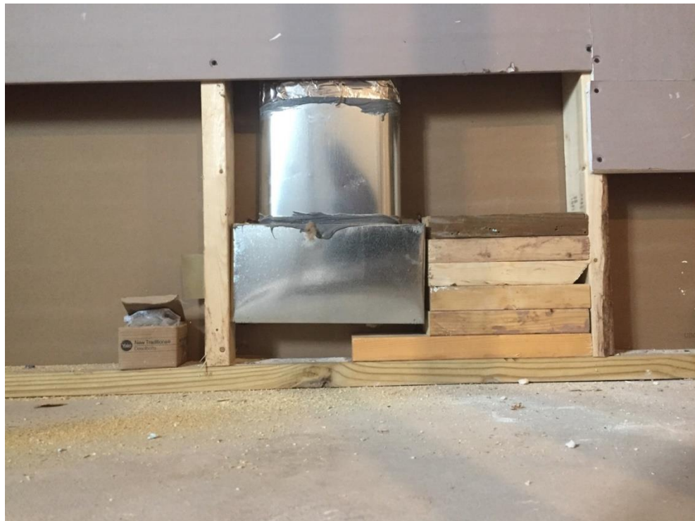
Figure 10-7. Cold Air Return Blocking.
