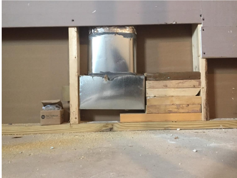
Figure 10-7. Cold Air Return Blocking.
