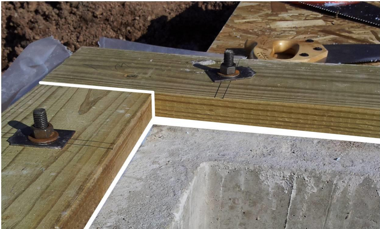
Figure 1-3. Sill Plate Installation.
