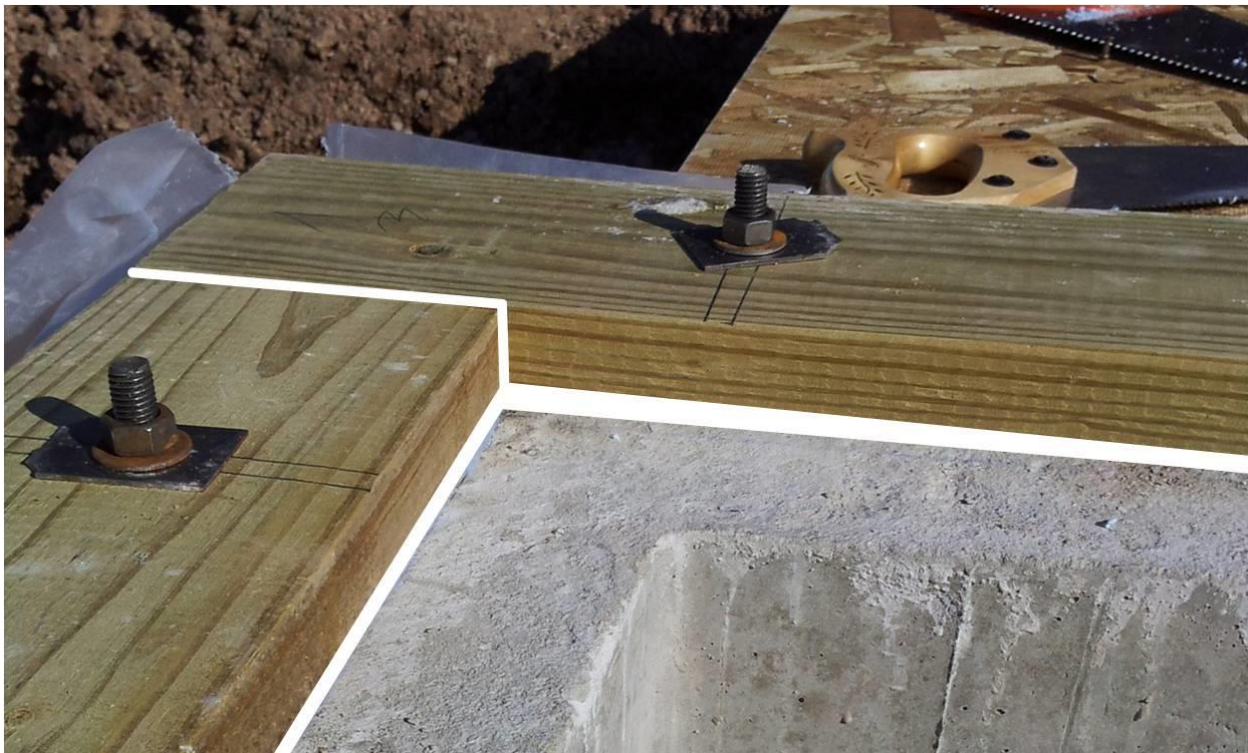
Figure 1-3. Sill Plate Installation.
